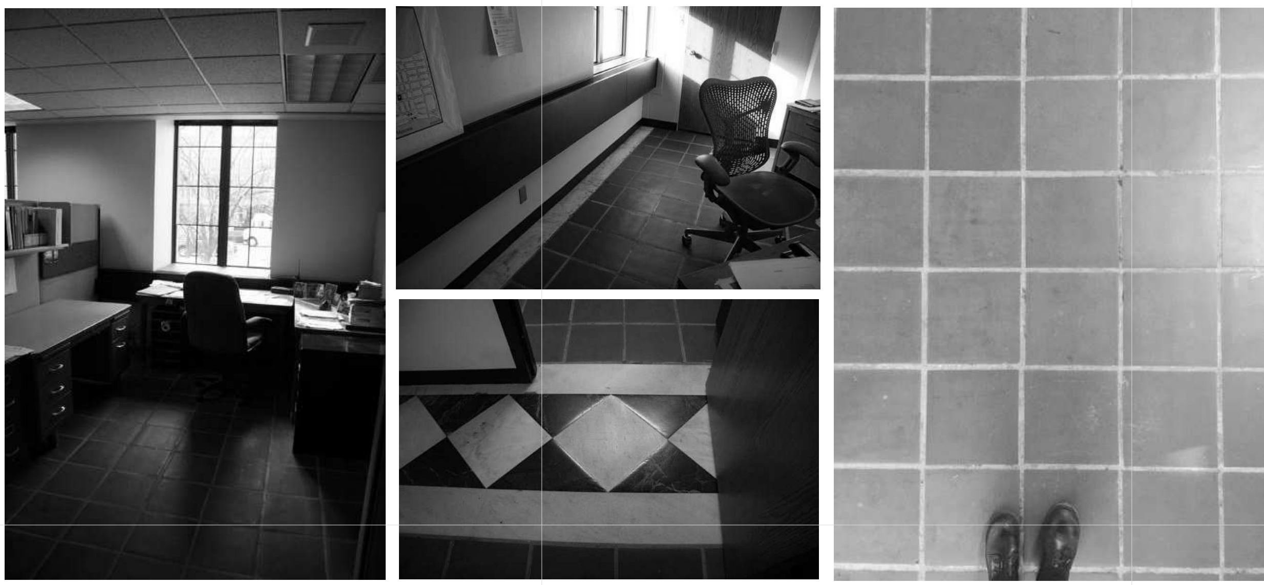
PHOTOGRAPHS OF EXISTING HISTORIC QUARRY TILE AT LEVEL 1, SOUTH OF GRID 2
