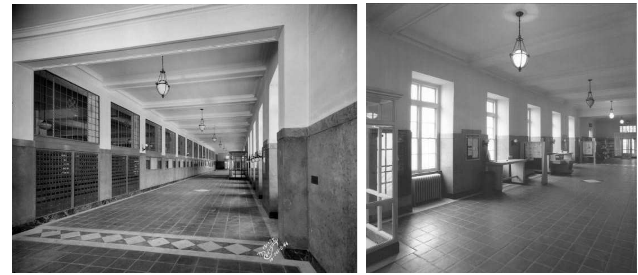
1920s PHOTOGRAPH OF THE ORIGINAL PUBLIC LOBBY AT LEVEL 1, LOOKING NE (ON THE LEFT), AND SW (ON THE RIGHT)
